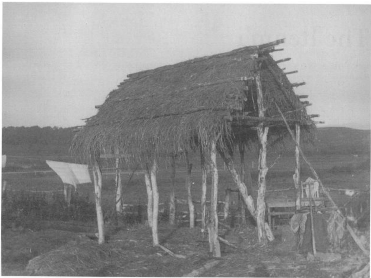
33 An Item'i storage house, pile-construction, Kovran village, September 1992. Photo: Victor A. Shnirelman.
